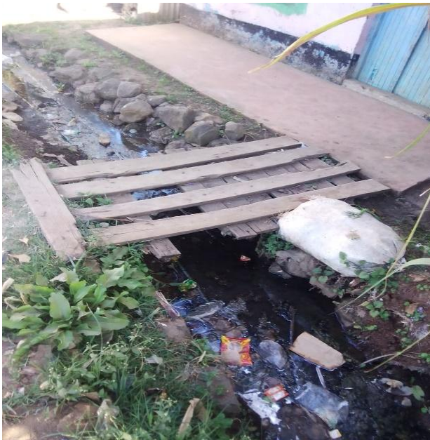
c) Open drain near a residential leading to Sewerage plant
